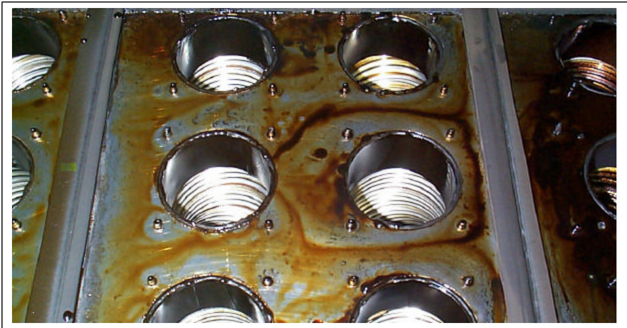
Figure 4: the same condenser tube after the self-cleaning cycle
